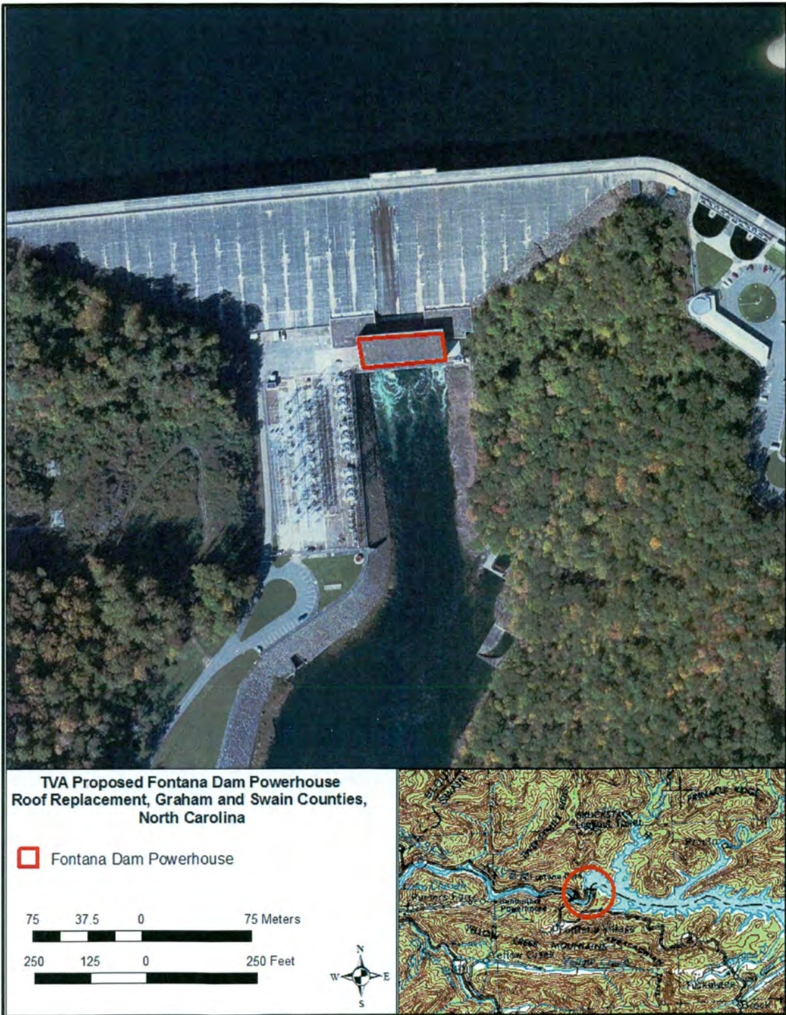
Figure 1. Aerial view of the Fontana Dam Powerhouse Roof.
