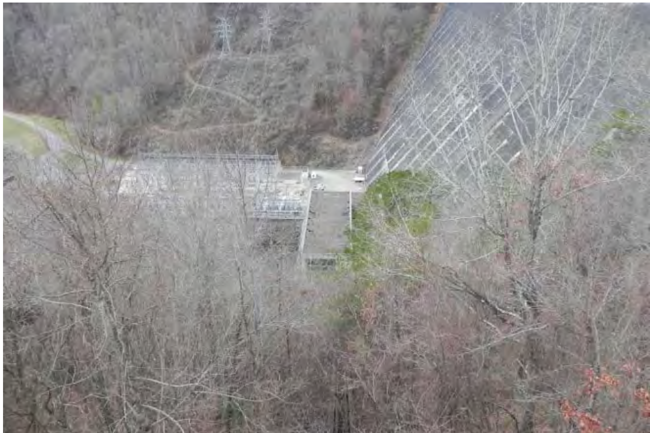
View of Power House roof from Visitor's Center
