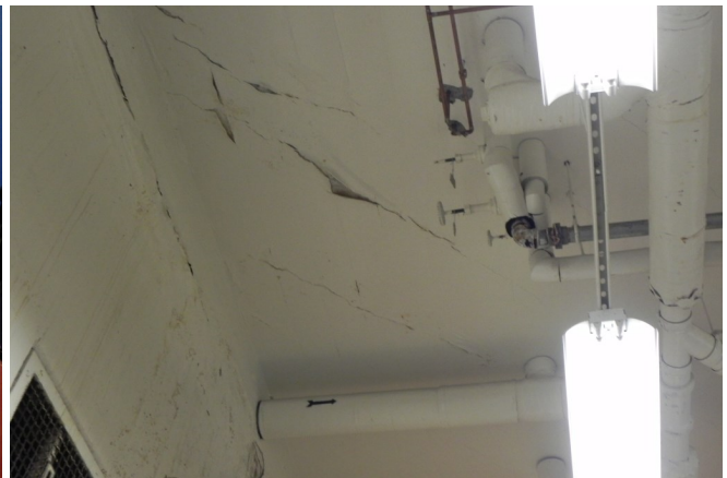
small parts storage (rear NE corner of building)
